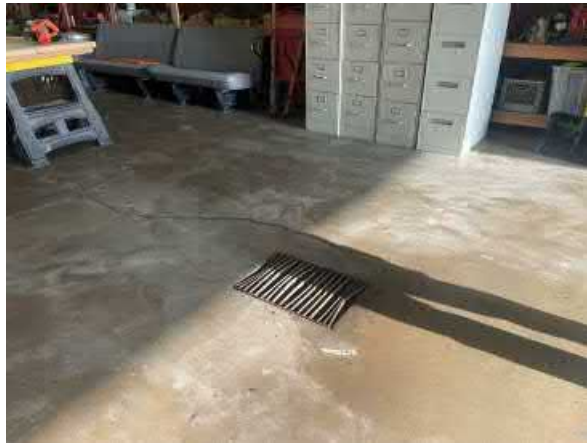
Photo #19 View of a stormwater drain located in the maintenance shop.
