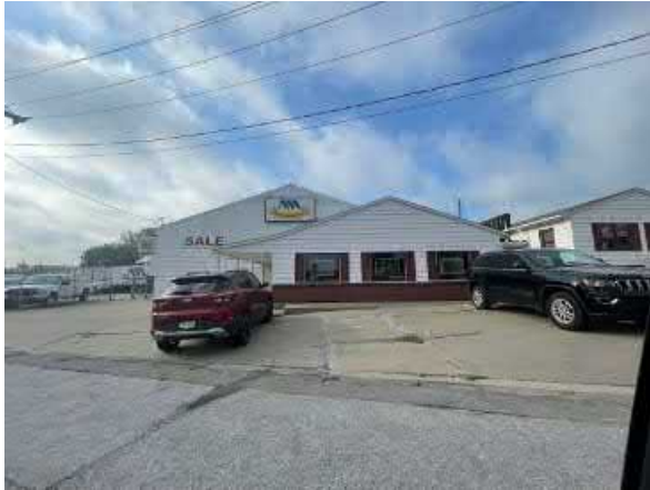
Photo #31 View of the east adjoining AAA Building Components, facing south.
