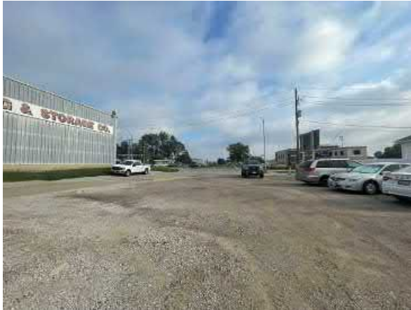
Photo #25 View of a gravel parking lot located on the east side of the front office.
