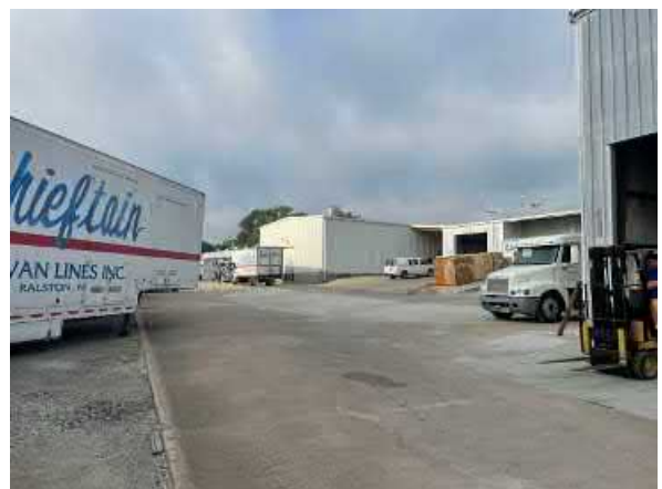
Photo #24 View of the loading/unloading area located on the east side of the storage warehouses.
