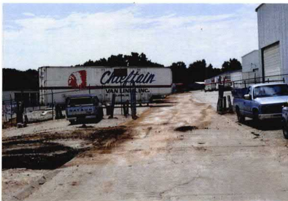
PHOTO 2. FACING SOUTH FROM WHERE FUEL ENTERED LOW AREA. PHOTO SHOWS PATH OF FUEL FLOW ALONG CONCRETE CURB. LEFT-HAND SIDE OF PHOTO SHOWS WHERE FUEL POOLED AND PERCOLATED INTO THE SOIL.
