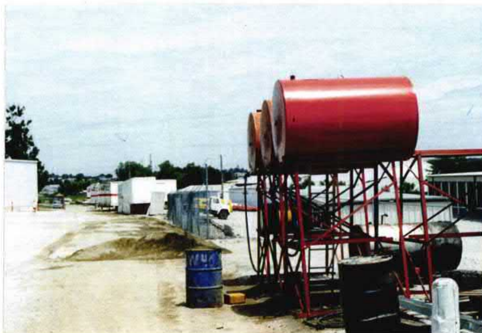
PHOTO 1. FACING NORTH FROM AREA OF ABOVE-GROUND TANKS. RELEASED FUEL TRAVELED NORTH OVER 400 FEET. DAMAGED TANK SAT FARTHEST SOUTH, AND HAS SINCE BEEN REPLACED. PILED SAND WAS USED AS AN ABSORBING MATERIAL.
