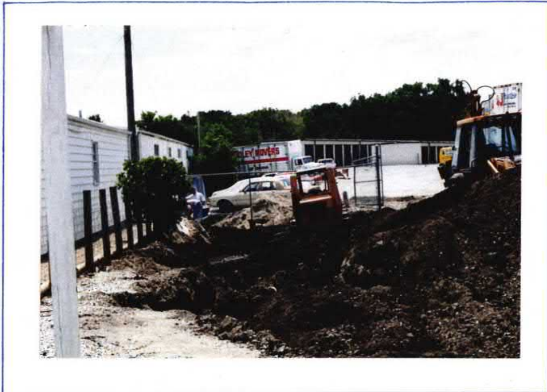
PHOTO 3. LOOKING SOUTH FROM NORTH END OF POOLED PRODUCT, WITH EXCAVATION OF MOST HEAVILY CONTAMINATED AREA IN PROGRESS. PHOTO SHOWS PORTION OF SAND DIKE USED TO PREVENT FURTHER SPREAD OF POOLED DIESEL.
