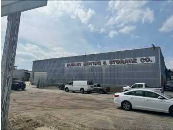
Photo #37 View of Chieftain Van Lines located west of the site. View from the east toward the west.
