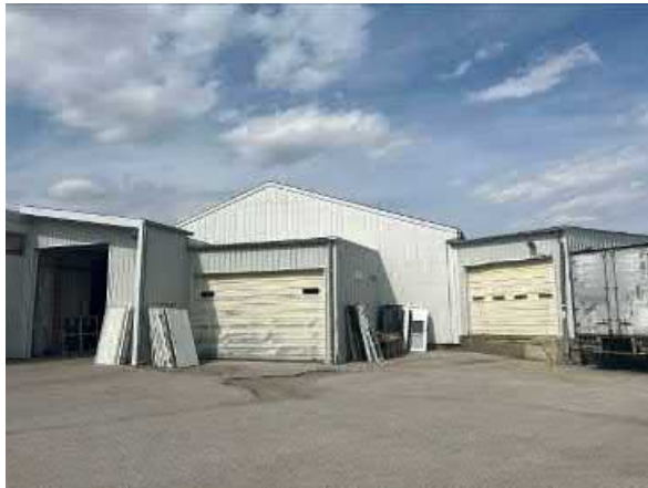
Photo #3 View of the eastern portion of the northern site parcel building. View from the east toward the west.
