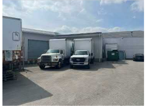
Photo #2 View of the northern portion of the northern site parcel building. View from the north toward the south.
