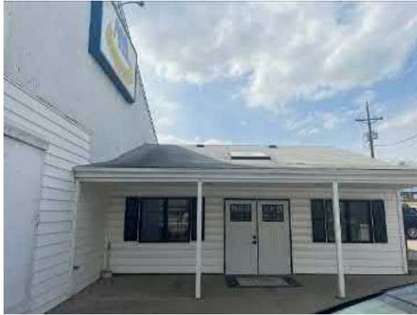
Photo #1 View of the show room and office area of the northern parcel site building. View from the east toward the west.
