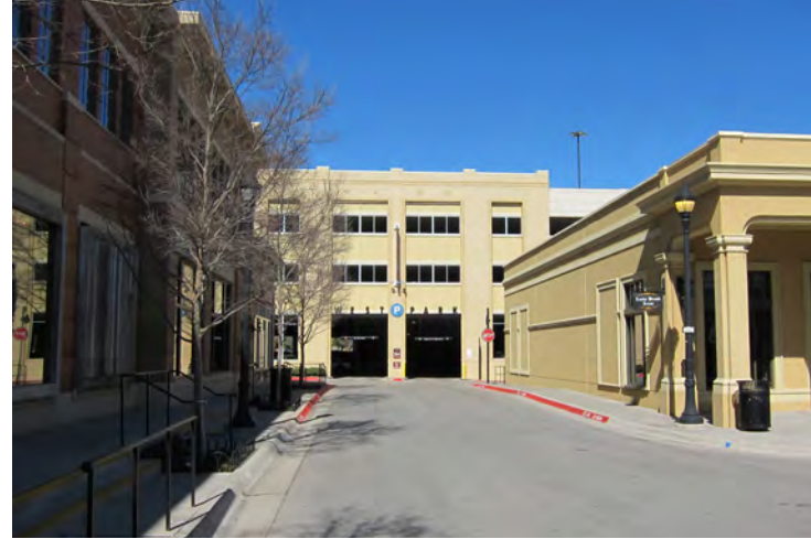
Interior Parking Structure
