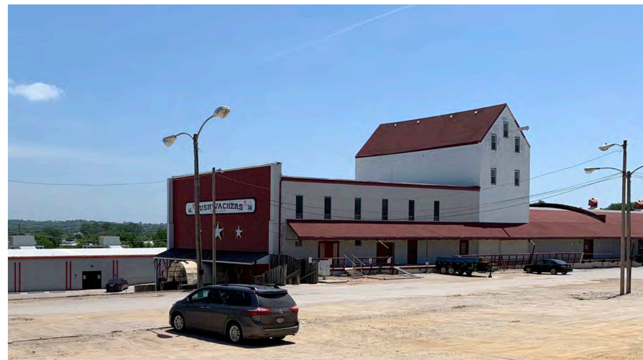
Granary existing conditions
