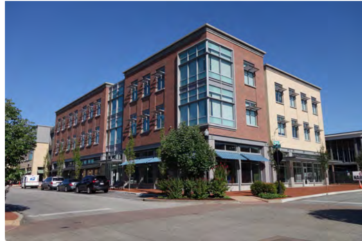
Three-Story Mixed-Use Building
