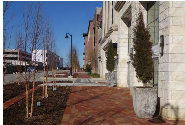
Example of a building with a small Setback
