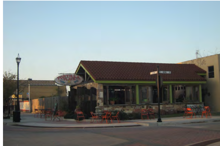
One-Story Retail Building
