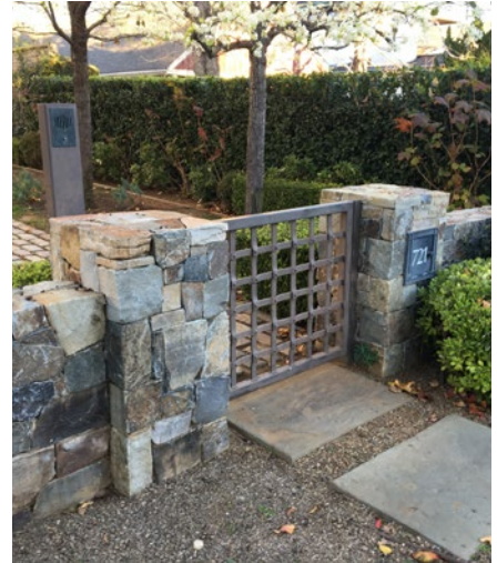
Stone screen wall with decorative metal gate
