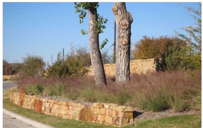
Terraced stone retaining walls
