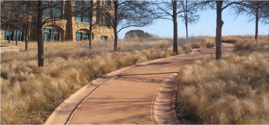
Colored concrete trail
