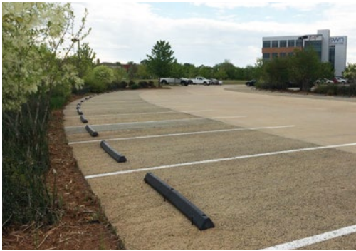
Surface parking lot with permeable pavement
