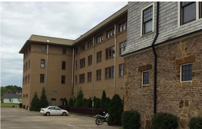
Rear landscape between parking lot and multi-family building
