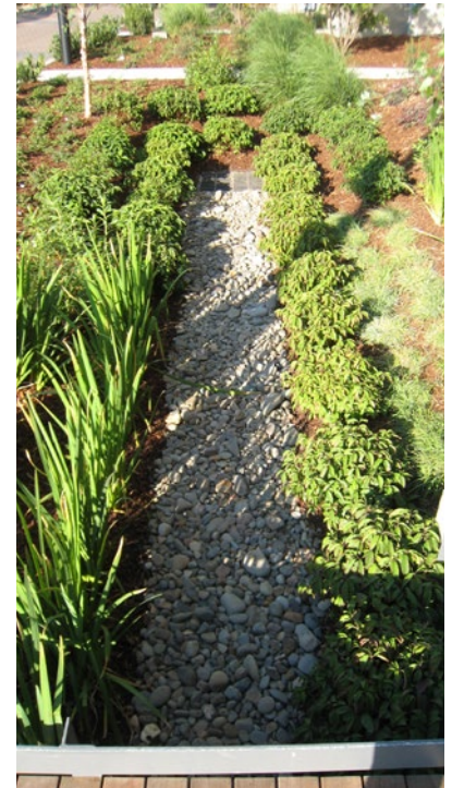
Dry creek bed and bioswale installation
