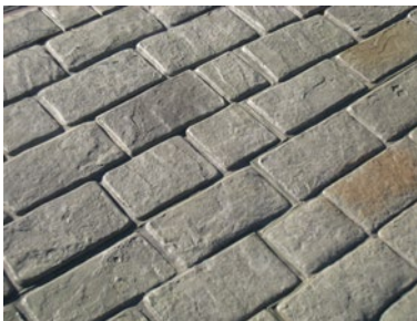
Stamped pattern in concrete
