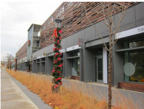
Parking structure with retail
