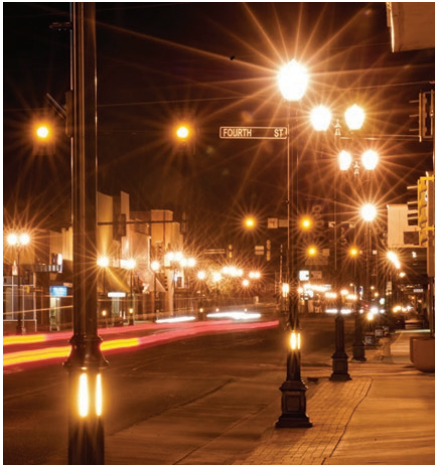
Glare caused by No Cutoff Fixtures
