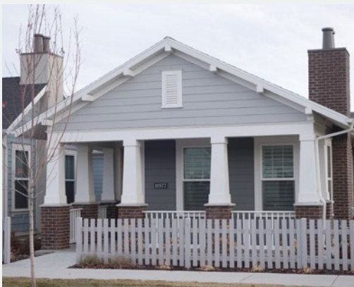
Front yard fence in front of cottage home
