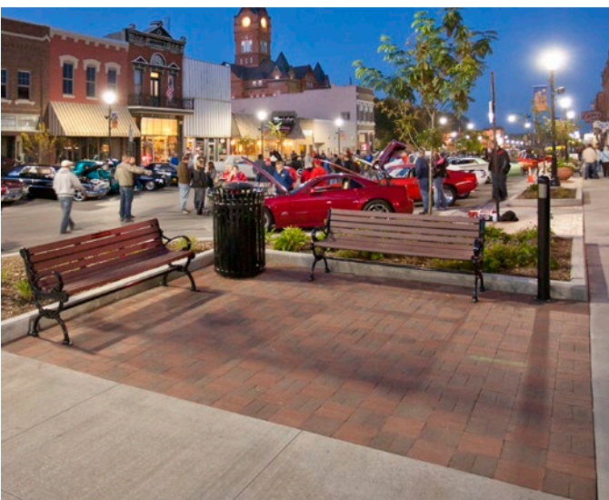
Clay pavers at streetscape node
